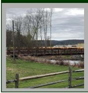
Description: Bridge specifically for use by pedestrians and bicyclists to cross a stream, water body, steep grade, or other existing feature. The design of the bridge should be based on anticipated users, including maintenance or emergency vehicles. Steel, fiberglass, and wood are
