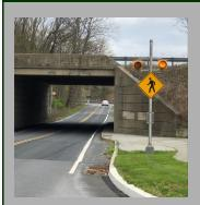
Description: A flashing warning device can be used in combination with pedestrian crossing signs and a marked crosswalk at uncontrolled crossing locations. Signs and flashing warning devices can be sidemounted or overhead. Additionally, flashing warning devices can be user activated. Rectangular Rapid Flashing Beacons (RRFBs) are one example of a flashing warning device.
