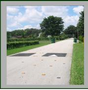
Description: Speed humps or speed tables that include wheel cutouts to allow larger vehicles to travel without slowing down to travel over the hump. They are intended to allow emergency vehicles or transit
