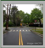
Description: A roundabout with a small diameter and traversable central island. Mini-roundabouts offer benefits similar to roundabouts, but with a smaller footprint and less cost. Mini-roundabouts are typically used in urban or small town settings on roadways with low speeds.
