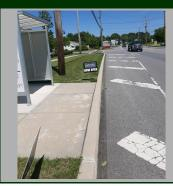
Description: A level loading area where the front, side, or rear door of a bus open to receive and discharge passengers. The clear area allows deployment of a front door ramp on the bus. The loading pad should be a firm and slip-resistant surface, such as concrete. Additionally, it should be free of conflicts, such as landscaping or street furniture. The
