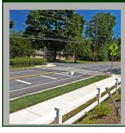
Description: Marked and elevated areas that are an extension of the sidewalk at mid-block locations or intersections. They can be used to increase pedestrian safety, calm traffic, and add to the community
