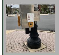
Description: Traffic signal equipment for pedestrians can include pedestrian pushbuttons, accessible pedestrian signals, passive detection for bicyclists or pedestrians, pedestrian signal heads, pedestrian countdown signal heads. Accessible pedestrian signals (APS) communicate information about the WALK and DON'T WALK
