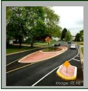
Description: A combination of special treatments used at the entrance to an area or neighborhood that alert drivers to slow down due to a change in environment. Gateway treatments can include signage to
